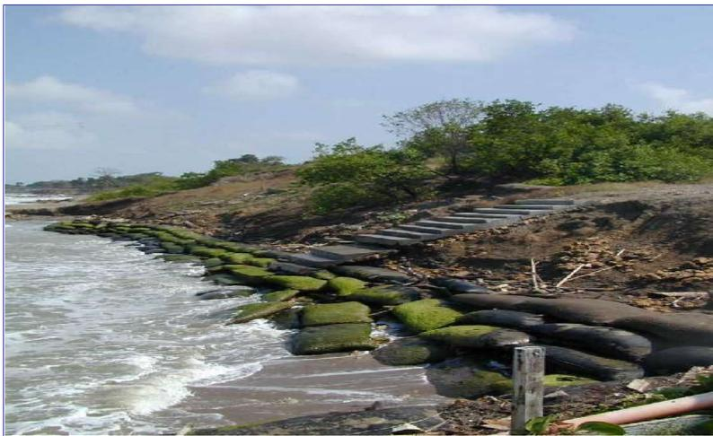
**Picture 11. Erosion caused by inadequate use of coastal defenses.**
